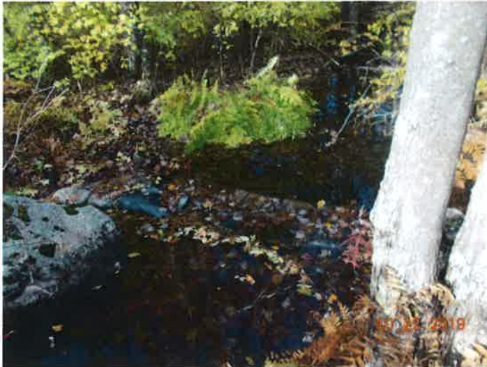
D183010 Harvey Lake Dam, Northwood, NH - Inspected October 22, 2019 DSCN2392
